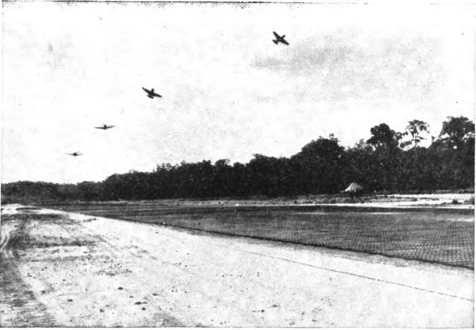
Figure 78. Pierced plank is the standard steel landing mat.
